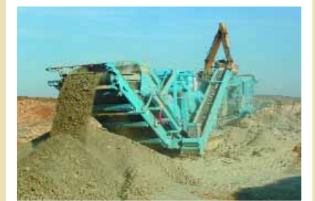
▲ 1180 Premiertrak working with a 4242SR to produce sub-base.
