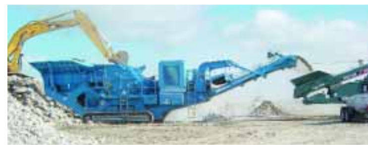
▲ 1412 Trakpactor feeding a Powerscreen Chieftain on a recycling application
